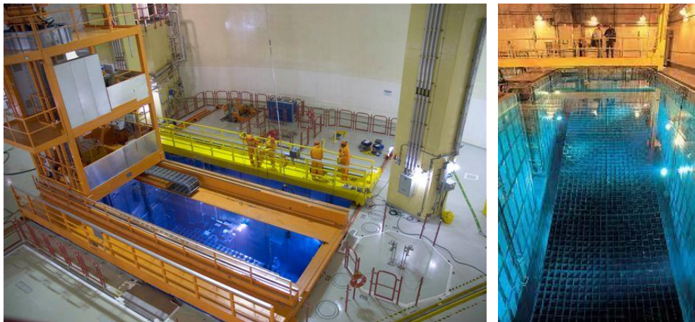
Figure 9 – Spent Fuel Pool of Angra 2 on the left and Angra 1 on the right
